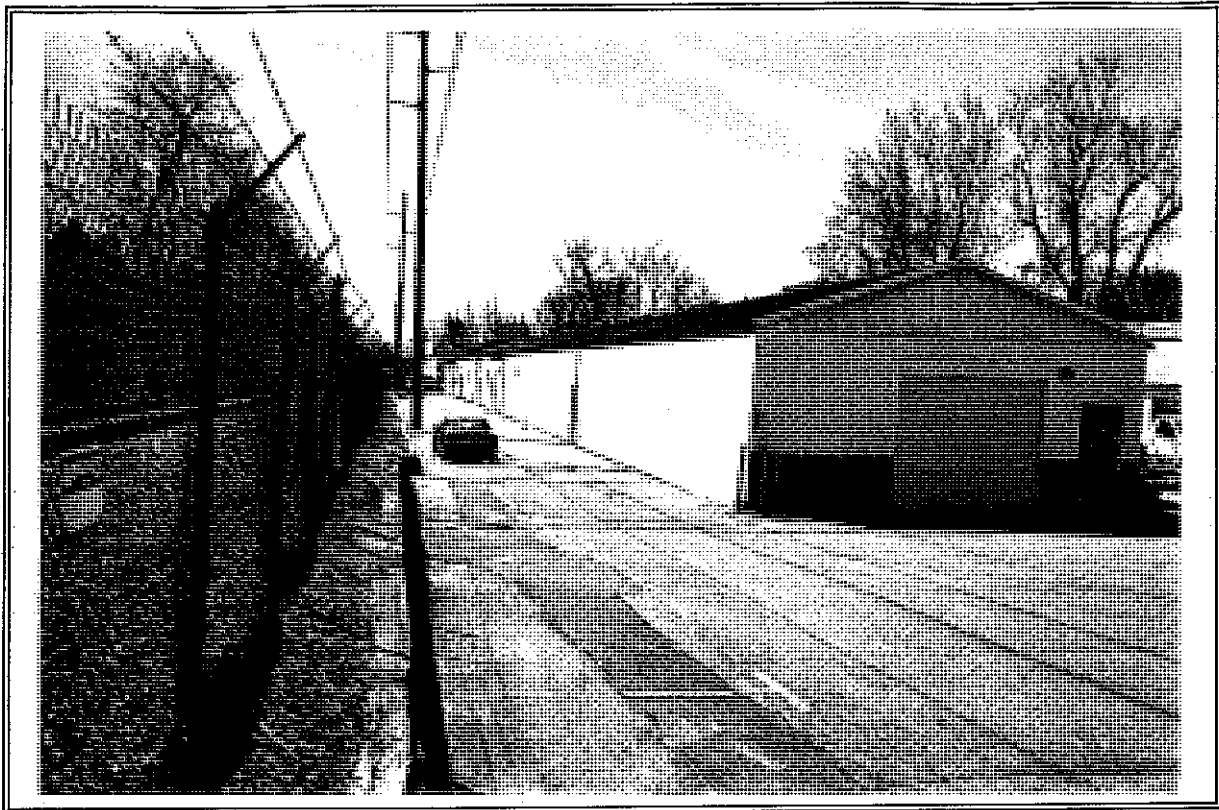
This shows the narrow space between Building 2 and the rail tracks. This view looks south.
