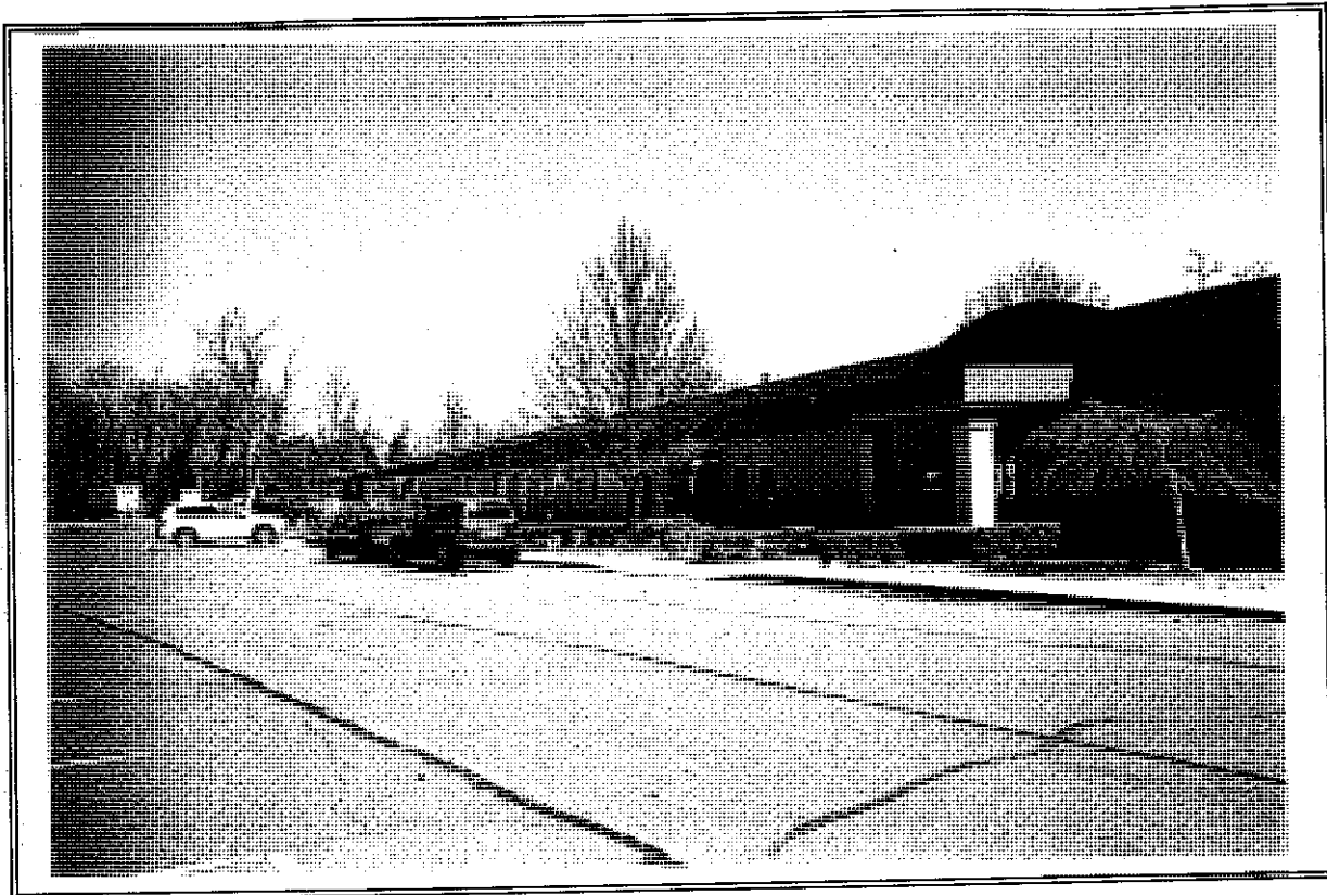
Building 7, at the building's south end, looking north.
