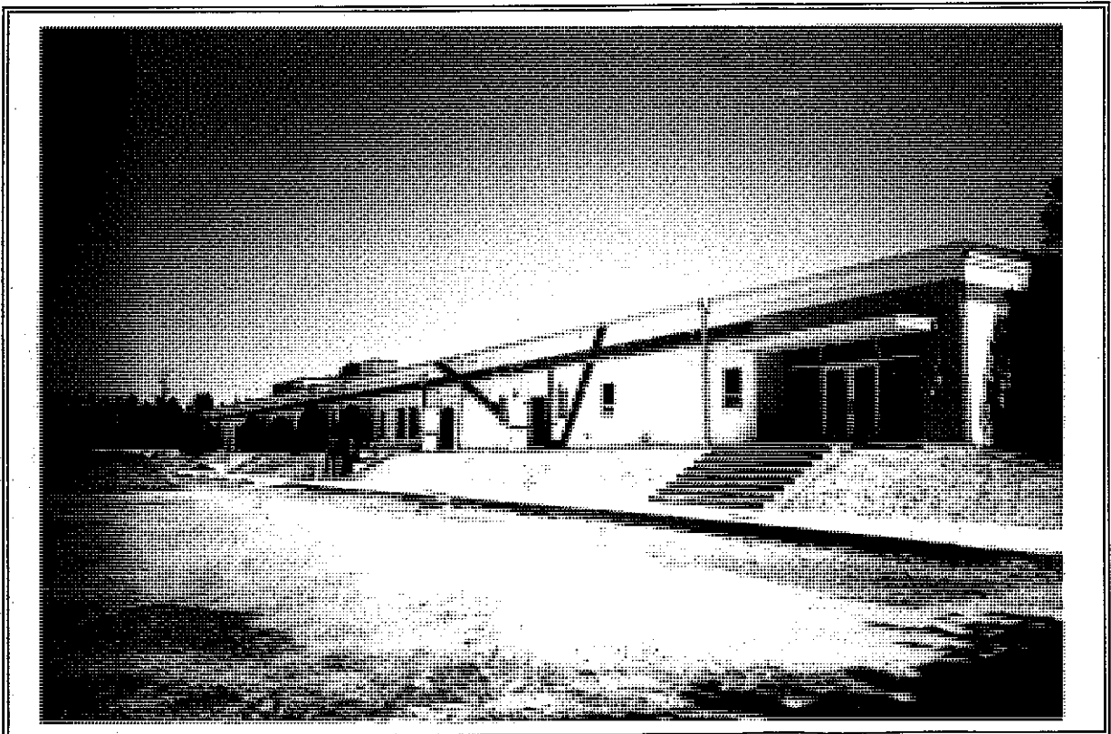
The west (front) wall of Building 17, undergoing renovation since the taking.
