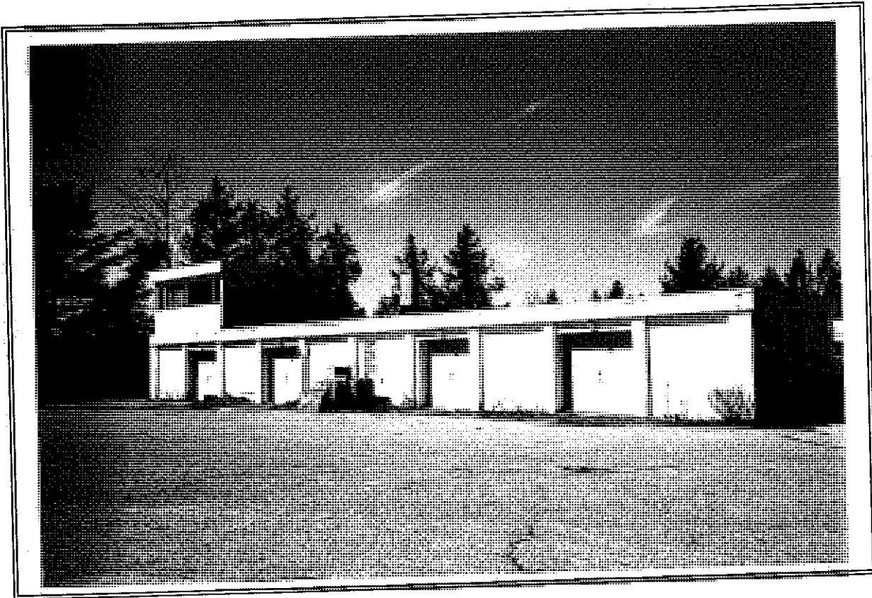
Building 18, facing southwest. This was appropriated.
