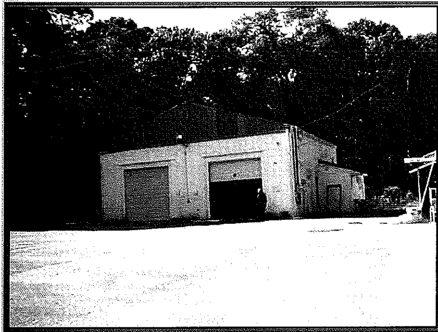
SUBJECT PROPERTY – IMPROVEMENTS SOUTH OF LIRR (TAKING AREA)
